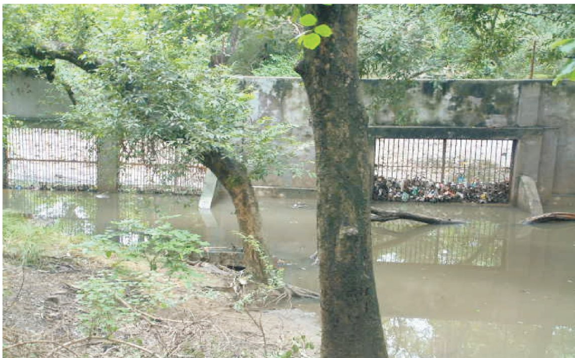
Figure V : Water inlets/ outlets - require proper maintenance
